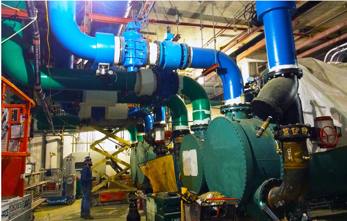
Central Chilled Water Plant Upgrades
